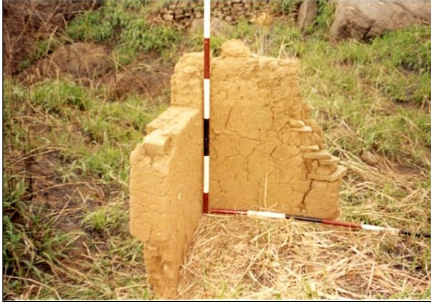
Fig. 9: A stone-mud wall (Photo by William N. Gblerkpor)
