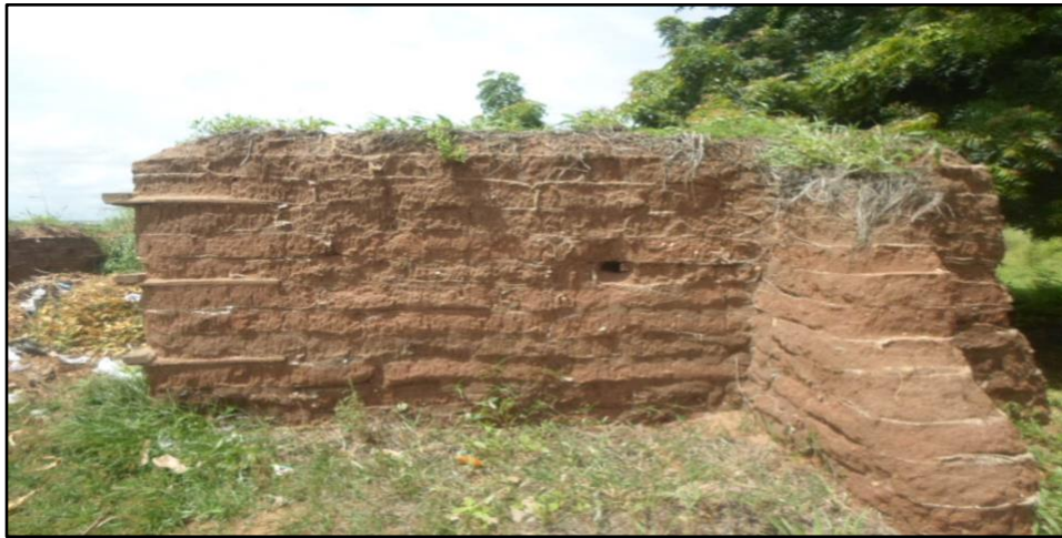
Figure 7. One of several abandoned vernacular structures at the ancient settlement quarter of Daazikessie. Note the vertical/horizontal bamboo posts within the coursed clay walls used to secure the superstructure in place (Photo: Author).
