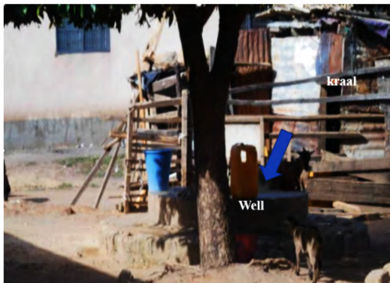
Figure 3 A hand-dug well with a kraal and animals besides the headwalls of the well
