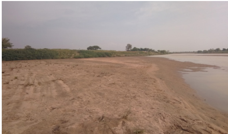
Figure 10 Siltation of Riverbed
