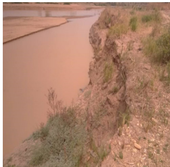
Figure 8 Scouring of the WVR resulting in gully formation
